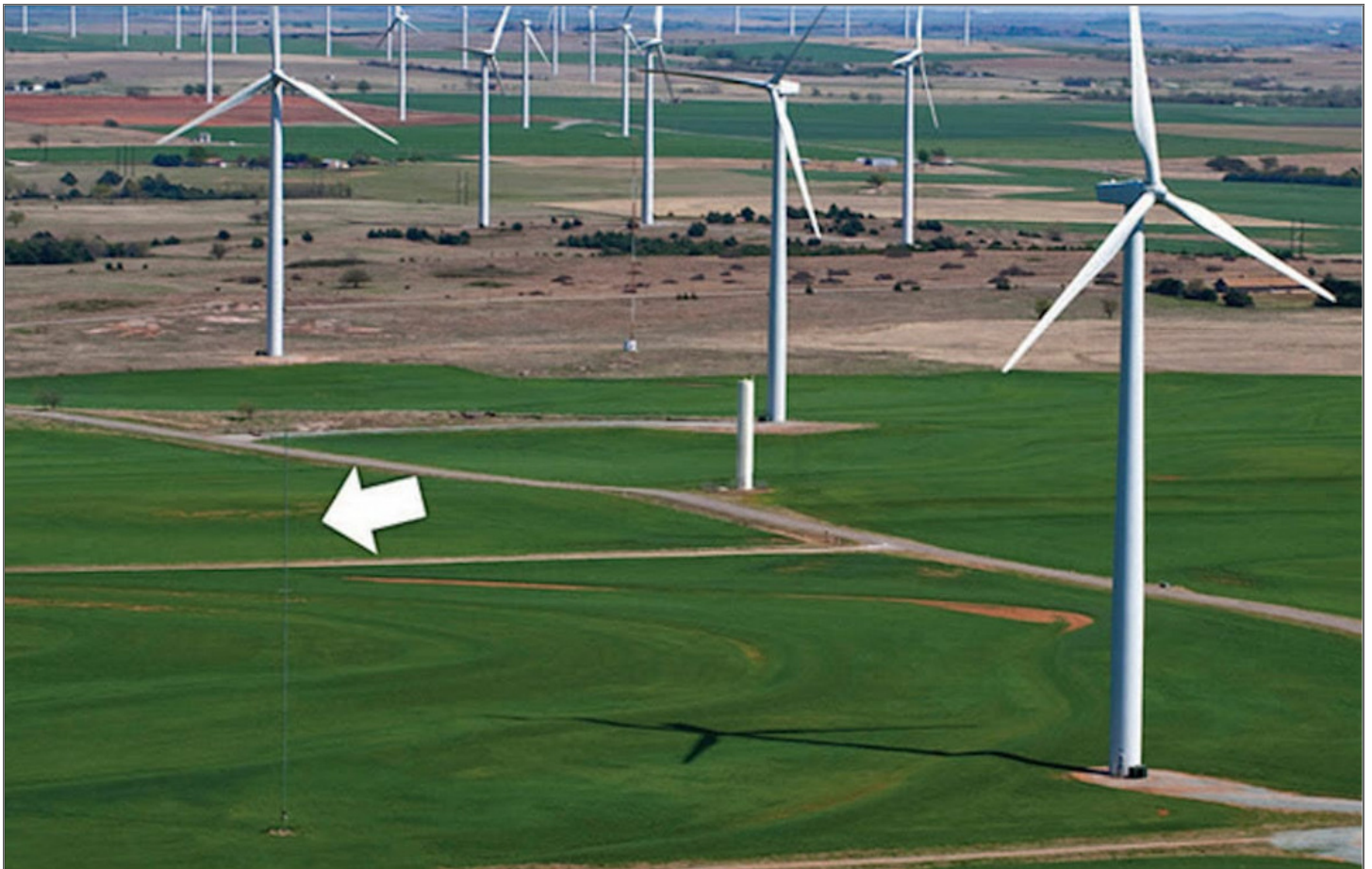
Unmarked meteorological evaluation towers must now be marked under new federal requirements. The arrow points out the almost invisible guy wires that pose such a risk to general aviation pilots.
